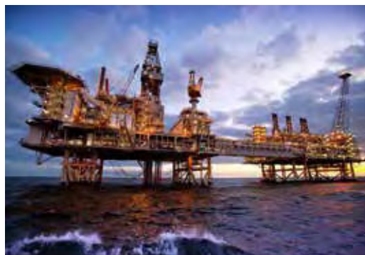
BP – West Azeri Platform - © BP Plc
